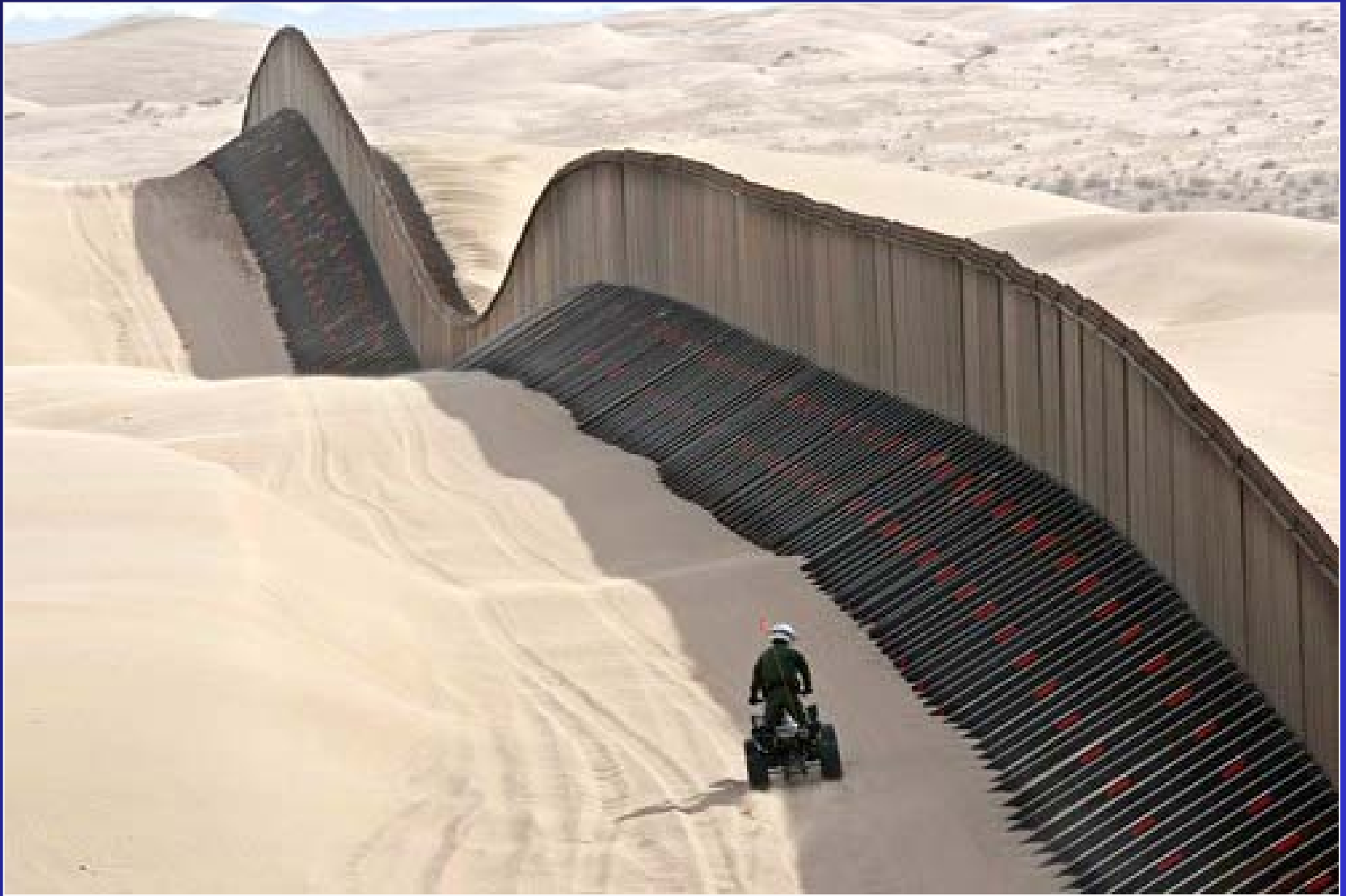
Border fence “floats” on sand dunes, Imperial Dunes, Calif.
