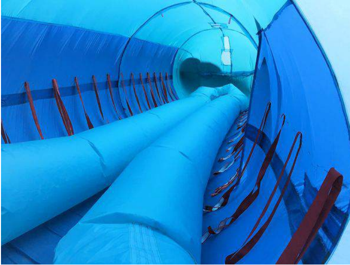
Airbeams fitted into a wing of the Ellipse.
