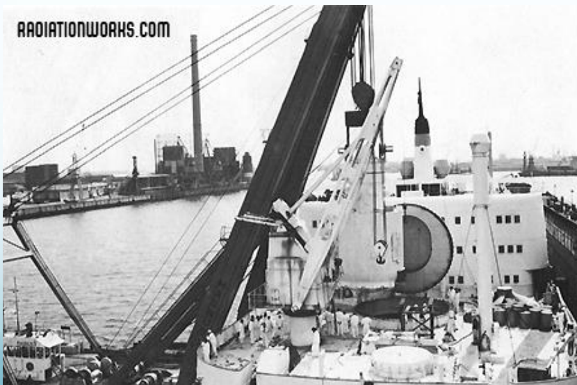
Above & bottom right: Removing the reactor during decommissioning. Source, three photos: http://www.radiationworks.com/ships/nsottohahn.htm
