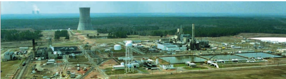
K Reactor with its new cooling tower, circa 1993. Vogtle nuclear power plant cooling towers are visible on the left horizon. Source: SRS Archives, negative 93-1340-17.
