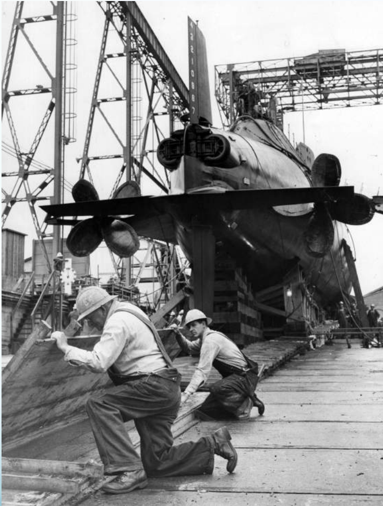
Note 4-bladed propellers and two aft torpedo tubes. Source, two photos: http://www.navsourc.org
