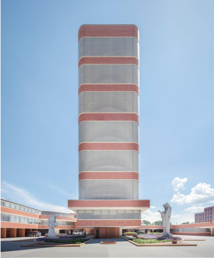
The SC Johnson Research Tower exterior & cross-section views. The taproot foundation extends 54 feet into the ground and the central core supports 15 cantilevered floors. Sources: (L) https://www.flickr.com/photos/88017382@N00/35847749345 (R) https://www.scjohnson.com
