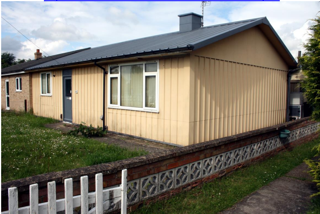
AW Hawksley BL8 semi-detached (duplex) aluminum bungalow in Cambridgeshire. Source: Jane Hearn, Prefab Museum
