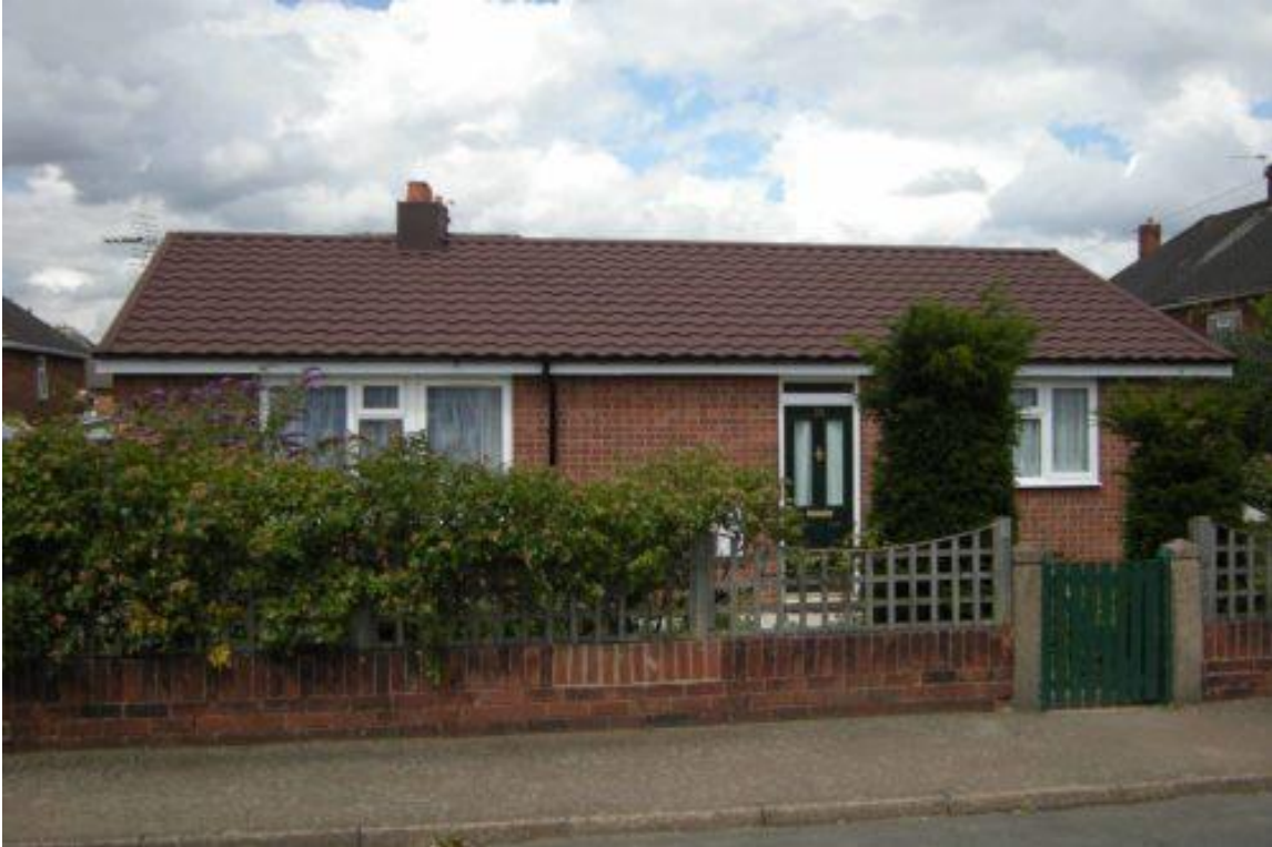
A refurbished AW Hawksley Bungalow with new brick veneer walls and lightweight steel roofing tile. Source: https://www.metrotile.co.uk/case-studies/hawkley-bungalows/
