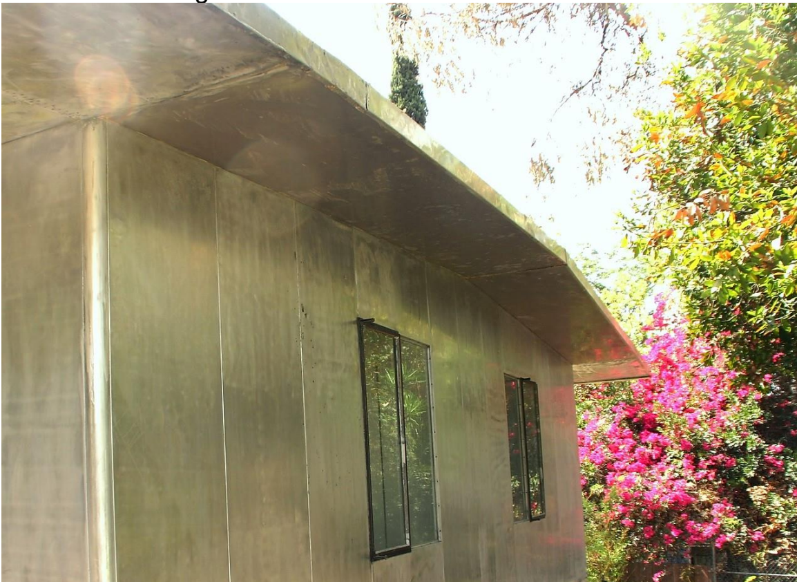
Restored aluminum exterior and roof overhang panels. Source: http://www.thefleethouse.com .
