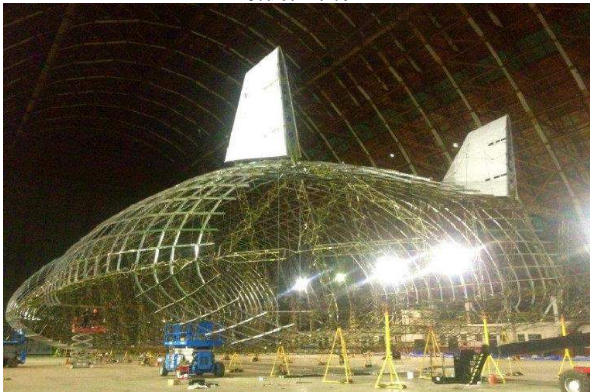
The Dragon Dream's assembled light weight, rigid aeroshell frame is installed around the internal main frame. Source: Aeros
