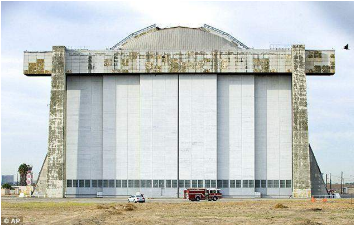
Part of the central roof of the North Tustin blimp hangar collapsed. Source: Associated Press via Daily Mail
