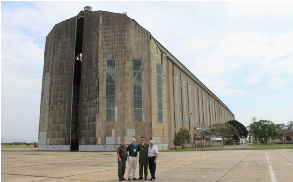
ADB airship hangar. Source: https://www.cbc.ca/news/ , 11 Mar 2018
