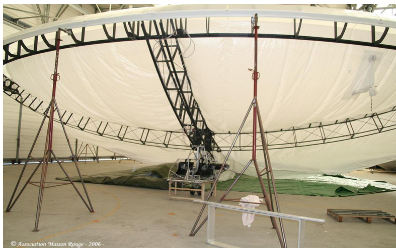
Alizé with its lower skin removed showing the internal rigid structures. Source: Association Moulin Rouge (2006)
