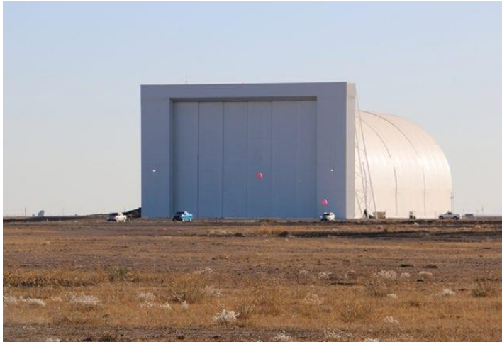
Sceye resumed flight operations at Roswell in 2020 after completing the hangar restoration. Source: Lisa Dunlap photo / Roswell Daily Record Online
