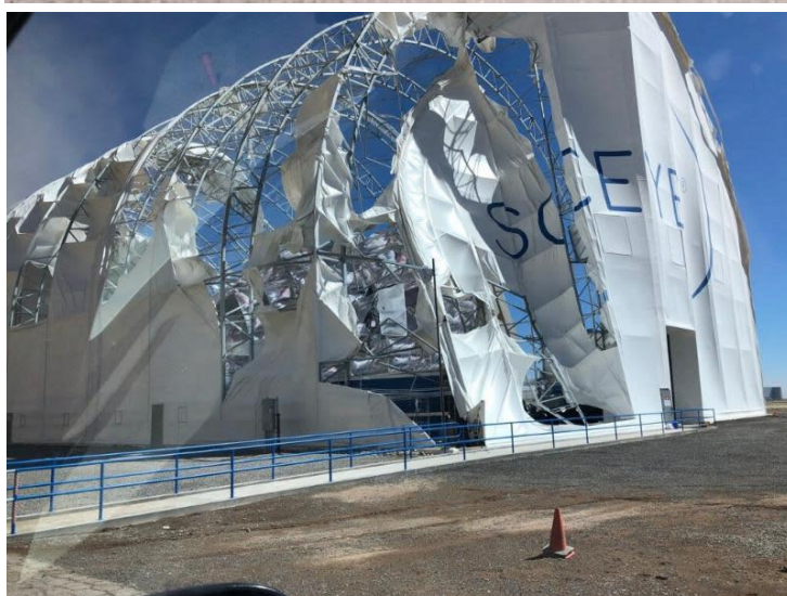
Damaged Roswell hangar after 12 March 2019 windstorm that also destroyed the 65 ft SSV. Source: Summit.com
