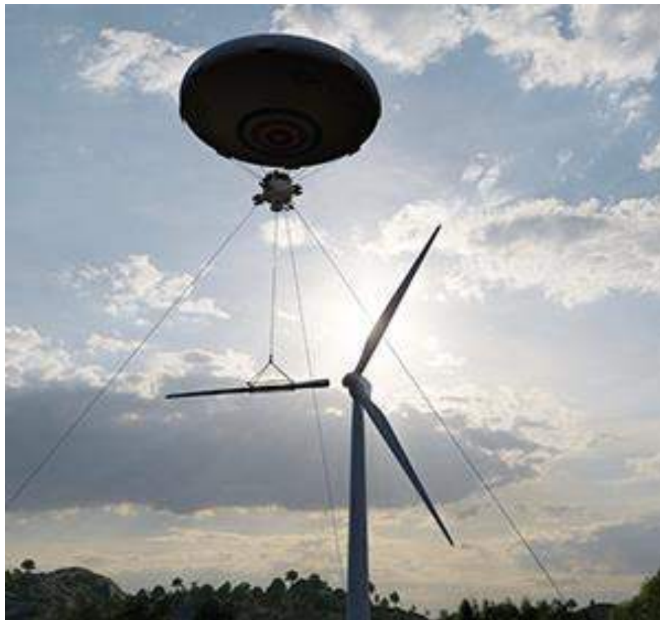
Rendering of a Sky Crane installing / removing a wind turbine blade. Note that the Sky Crane is tethered at three points for added stability during this high-precision evolution. Source: SkyLifter
