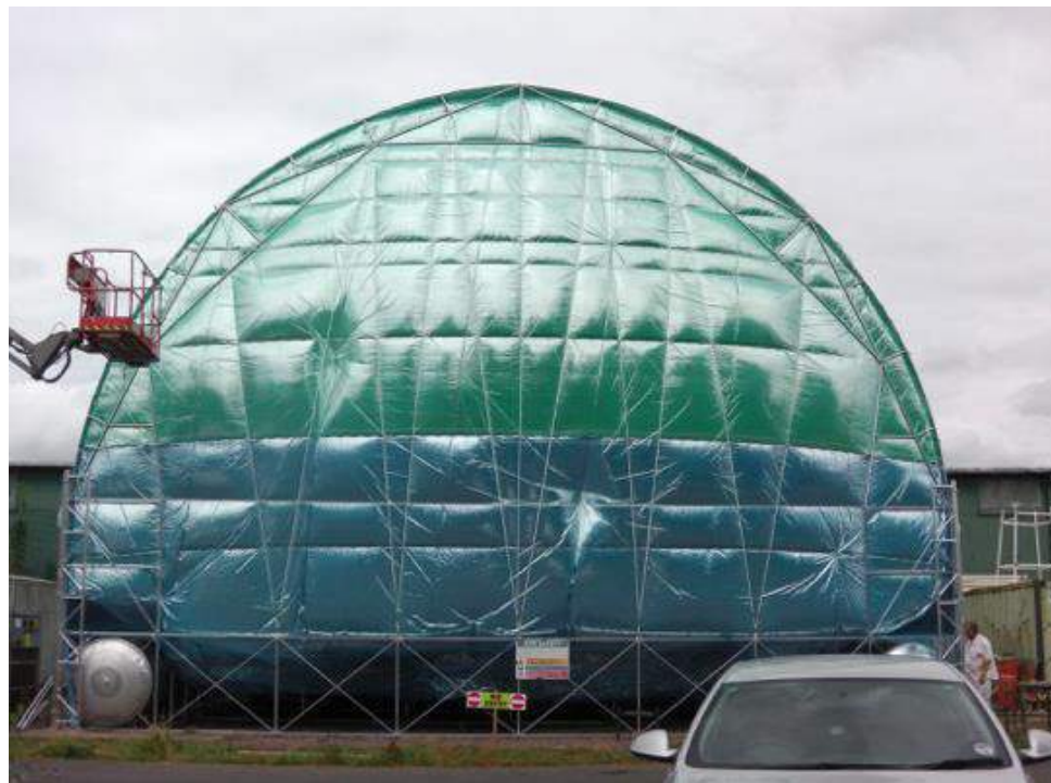
Gas envelope installed in one variable lift unit. Source, both photos: Varialift.
