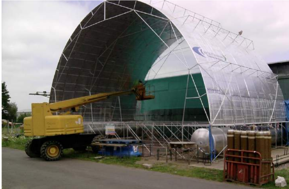
Aluminum shell complete on one variable lift unit.
