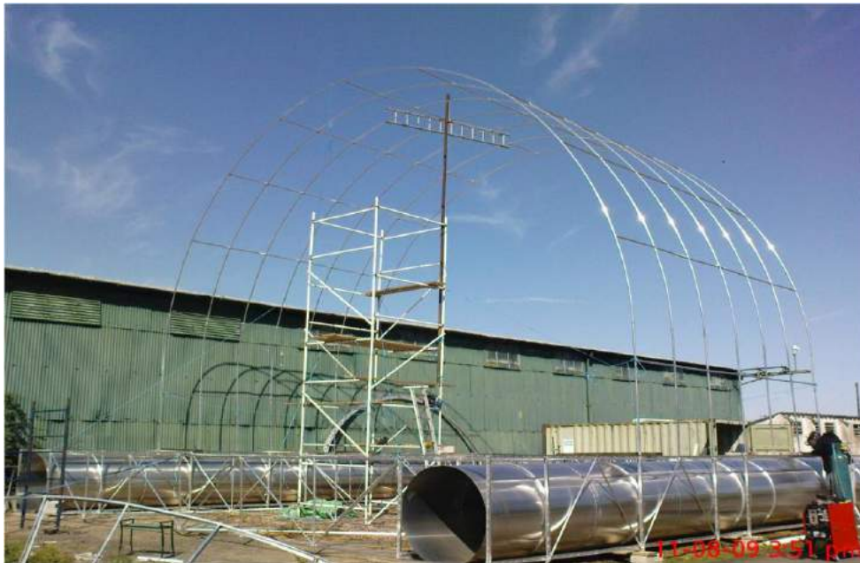
Start of the tubular framework for one variable lift unit showing the positions of the two receiver tanks. Source, both photos: Varialift.
