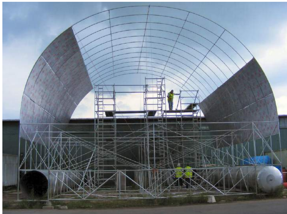
Installation of aluminum skin on a variable lift unit in progress. Source, both photos: Varialift.
