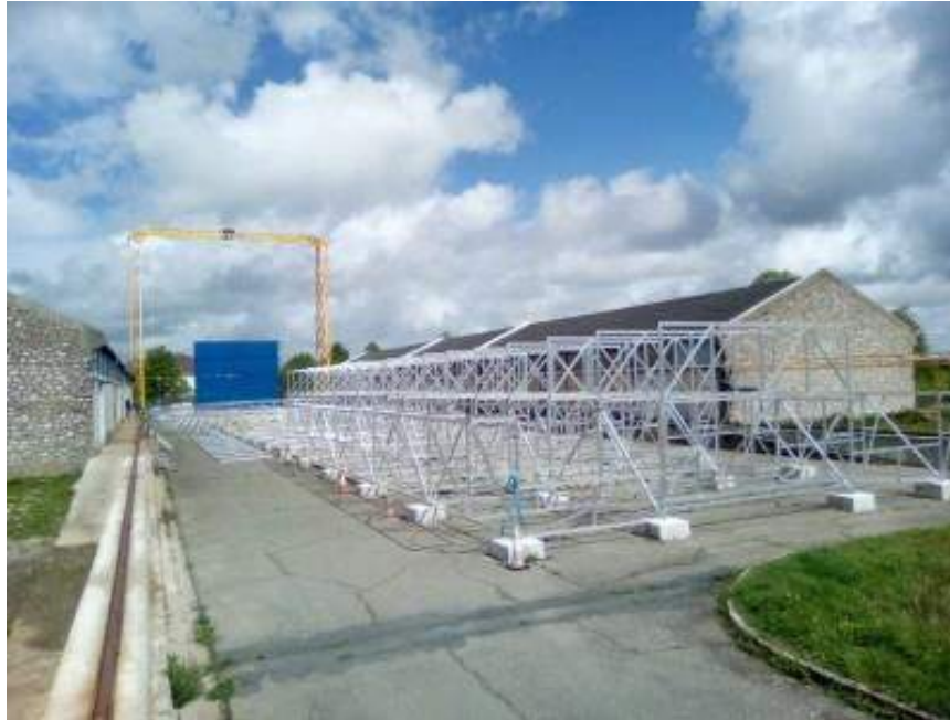
New gantry crane installed and construction started on the cargo bay for the first ARH-PT airship. Note that the first five modules of the cargo bay have been completed and are sitting on their assembly foundations. Source: Varialift (circa mid-2019)
