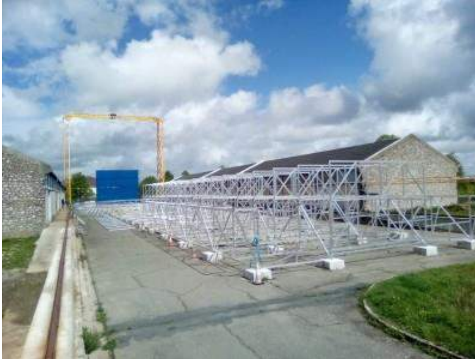
Construction started on the cargo bays. Source: Varilift
