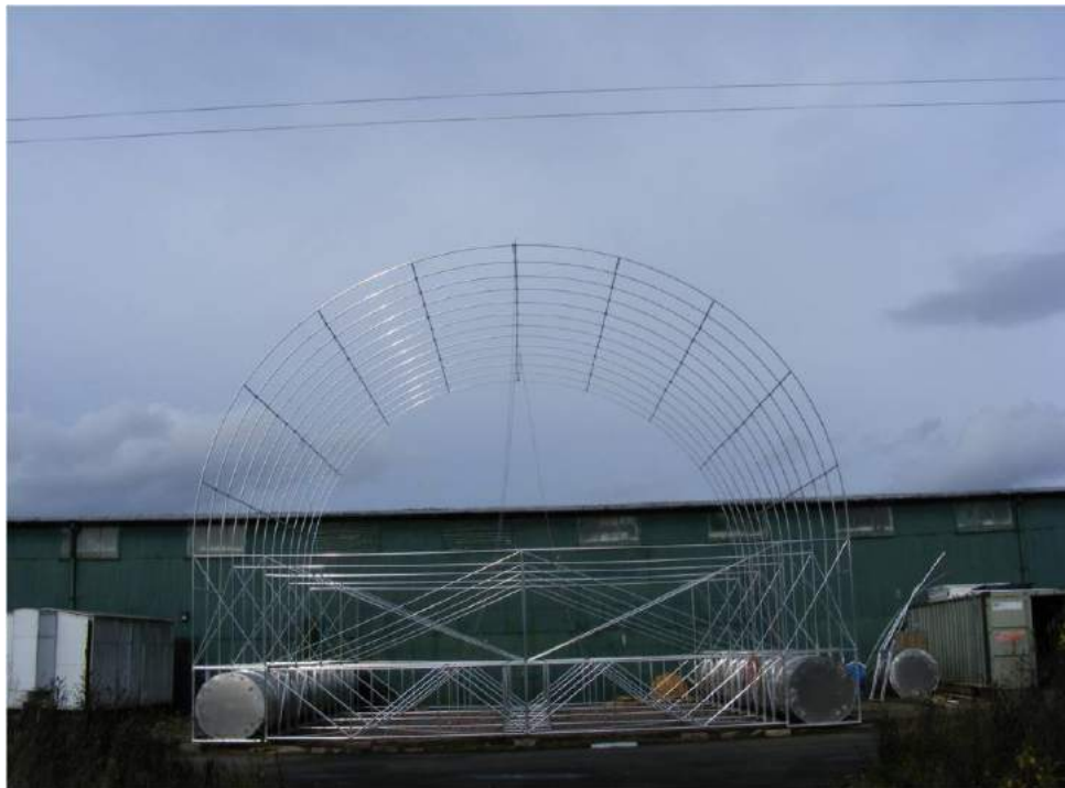
Tubular framework for one variable lift unit nearing completion. Source: Varialift.
