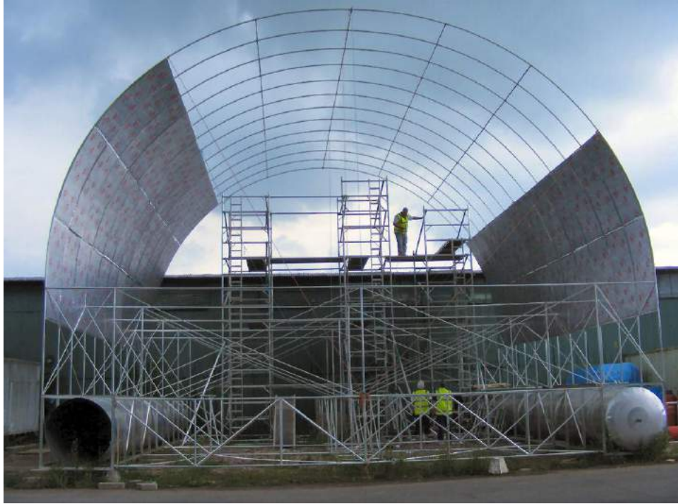
Installation of aluminum skin on a variable lift unit. Source: Varialift.
