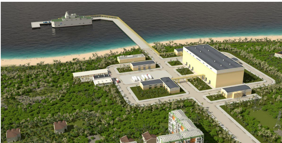
Rendering of an OPEB at a tropical site. Source: Strana_Rosatom Aisberg claims that the OPEB announced in January 2021 can operate in tropical and subtropical climates, with seawater temperatures up to 40°C (104°F) and outside air temperatures up to 47°C (117°F).
