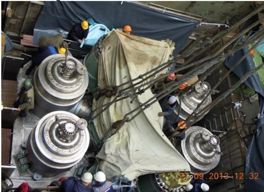
(Above) KLT-40S modular primary system being installed on Lomonosov. (Below) KLT-40S in place with a tarp over the reactor vessel and four main circulation pumps. The four steam generators are visible. Source: Barents Observer
