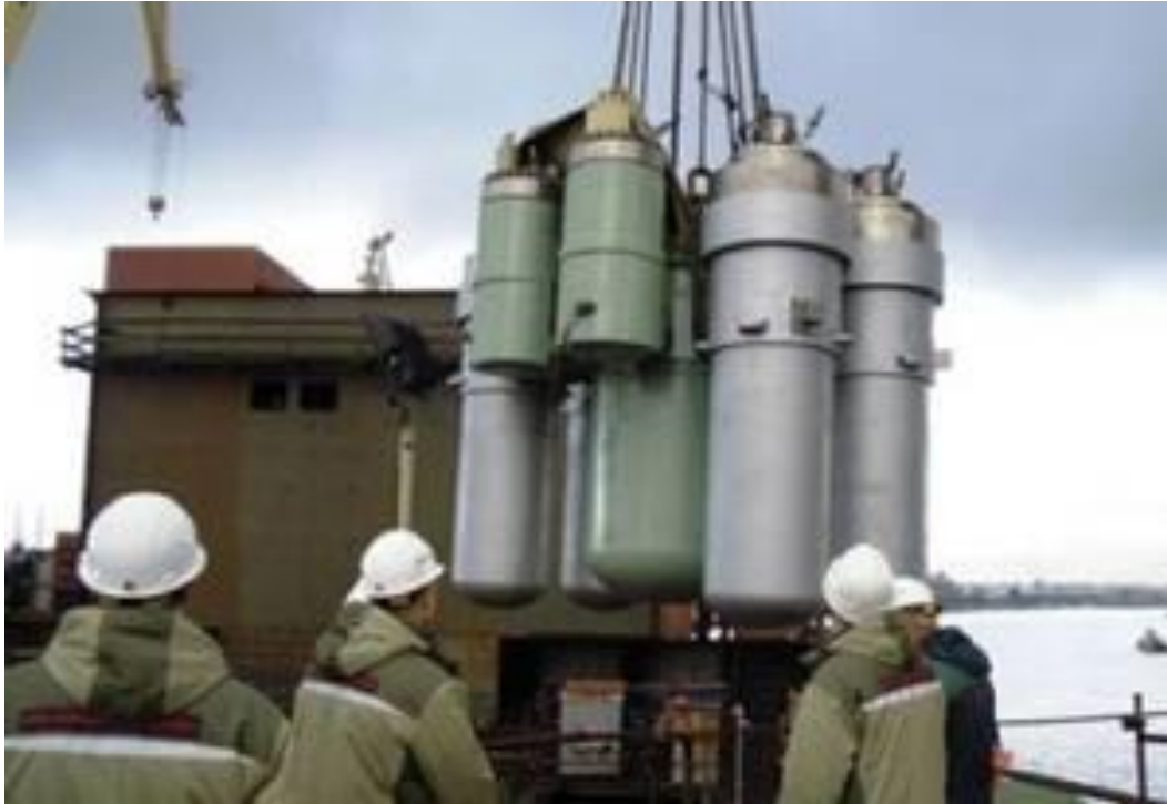
(Above) KLT-40S modular primary system being installed on Lomonosov. (Below) KLT-40S in place with a tarp over the reactor vessel and four main circulation pumps. The four steam generators are visible. Source: Barents Observer
