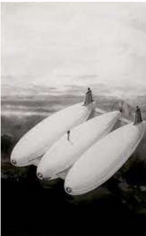
Above: Aereon III at Mercer County Airport, Trenton, NJ, 1964. Note the 21-foot (6.4-meter) diameter, two-bladed helicopter rotor used as a propeller. Persons in the photo are C.A. Beck, J.R. Fitzpatrick, and M. Drew, Jr. (L to R). Source: "The Dynairship," by William McElwee Miller, Jr.
