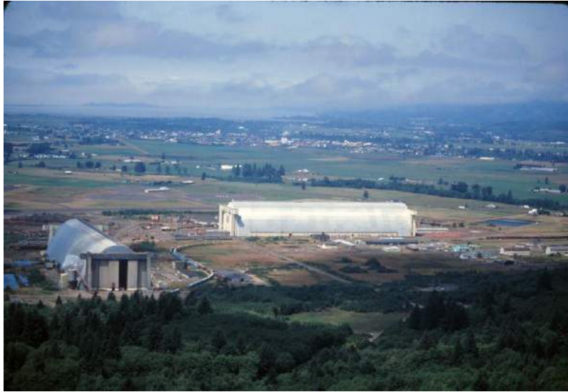
The AeroLift facility in Tillamook, OR. Source: Rob Crimmins
