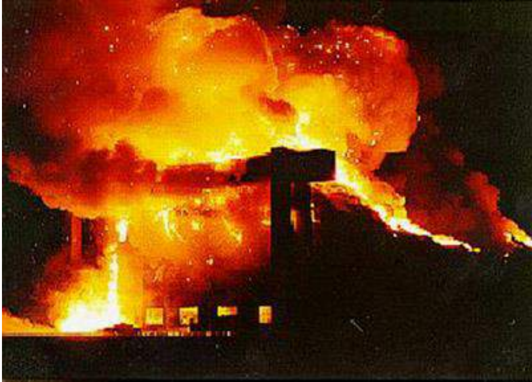
Airdock #2 engulfed in flames, 3 August 1995.
