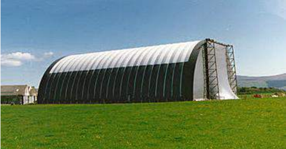
The AAC airship shed at Jurby, Isle of Man, was officially opened on 14 June 1988 and demolished 2009. Source: Airship Heritage Trust
