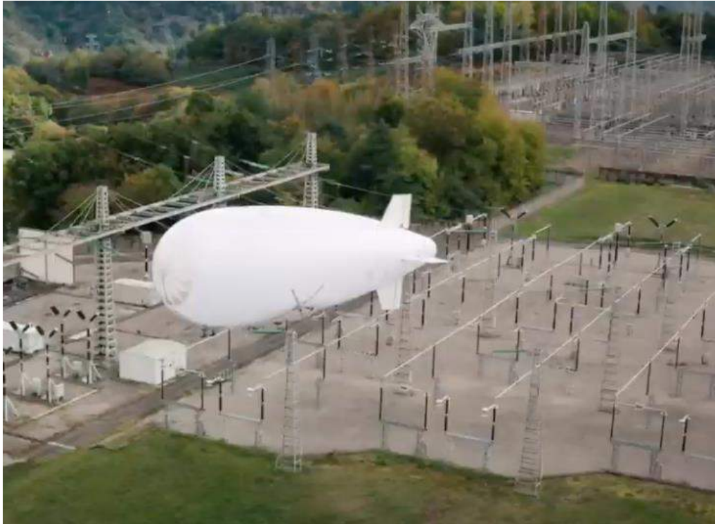
Diridrone flying over an RTE switchyard.
