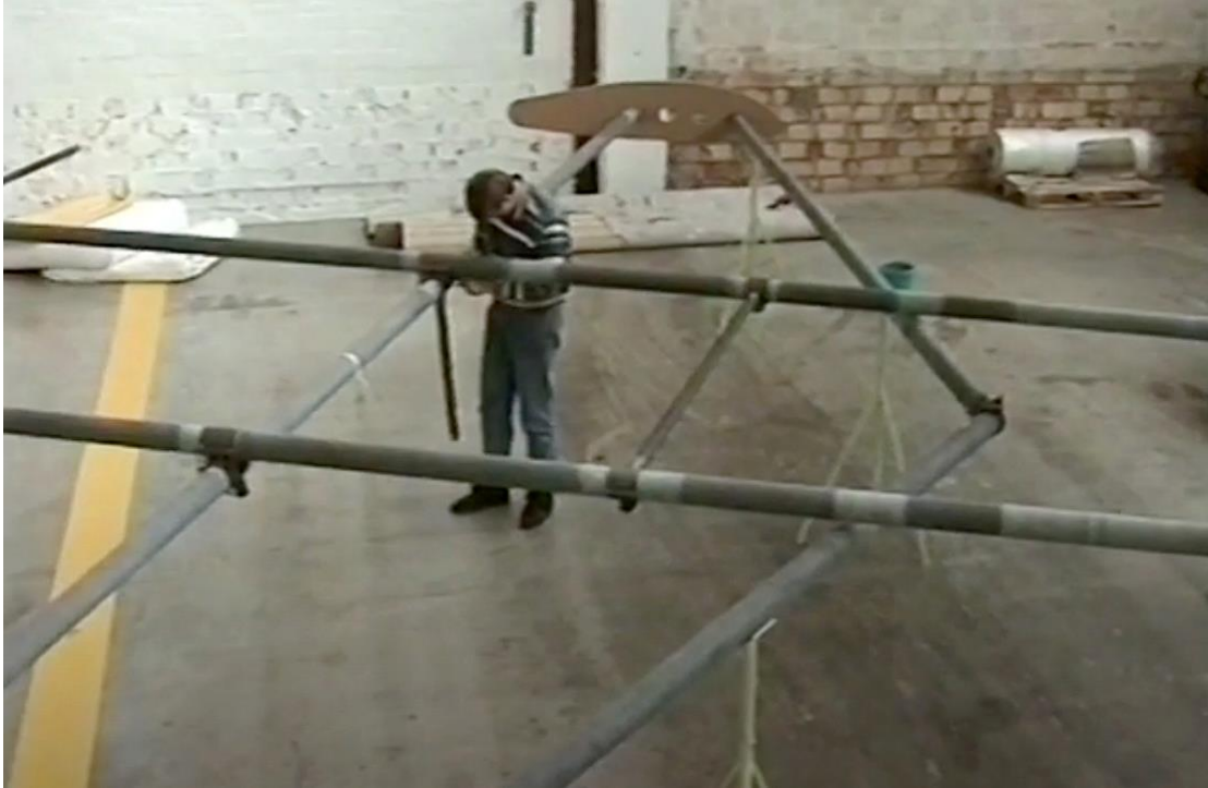
Mechanically-joined wing spars (with endplate in the background) and longerons, with vertical supports for the gondola being installed.
