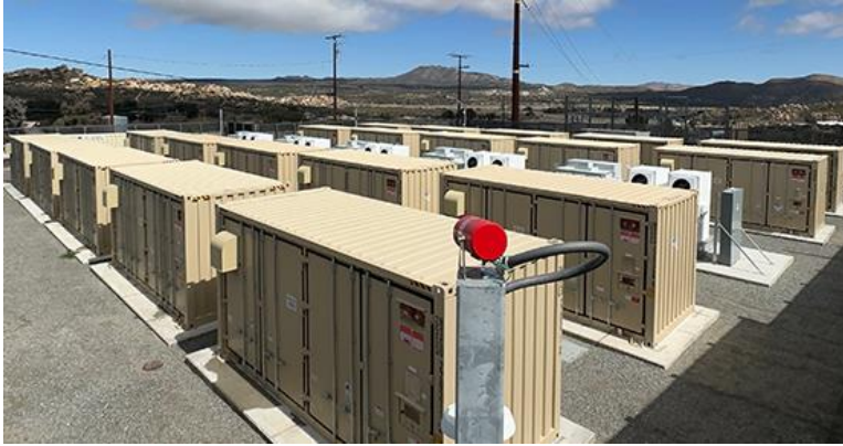
Boulevard Microgrid and Battery Energy Storage System Project uses Lithium iron phosphate (LFP) battery cells that have enhanced safety and fire prevention features. Source: SDG&E
